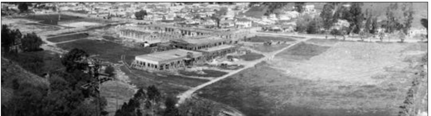
The school under construction in the "Happyland" district in 1927, the football field to the right, Yosemite Park to the left.
